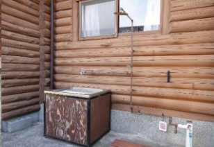
Outdoor sink and shower
